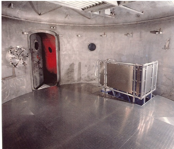
FIGURE 21. Upper level of the S-18 Altitude Chamber during renovation to serve as the Controlled Environment Research Chamber (CERC). NASA Photo.
